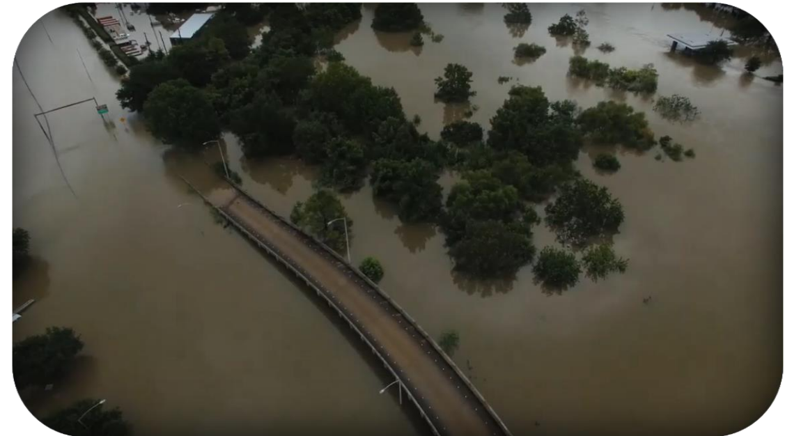
Compound flooding in Houston, TX.
