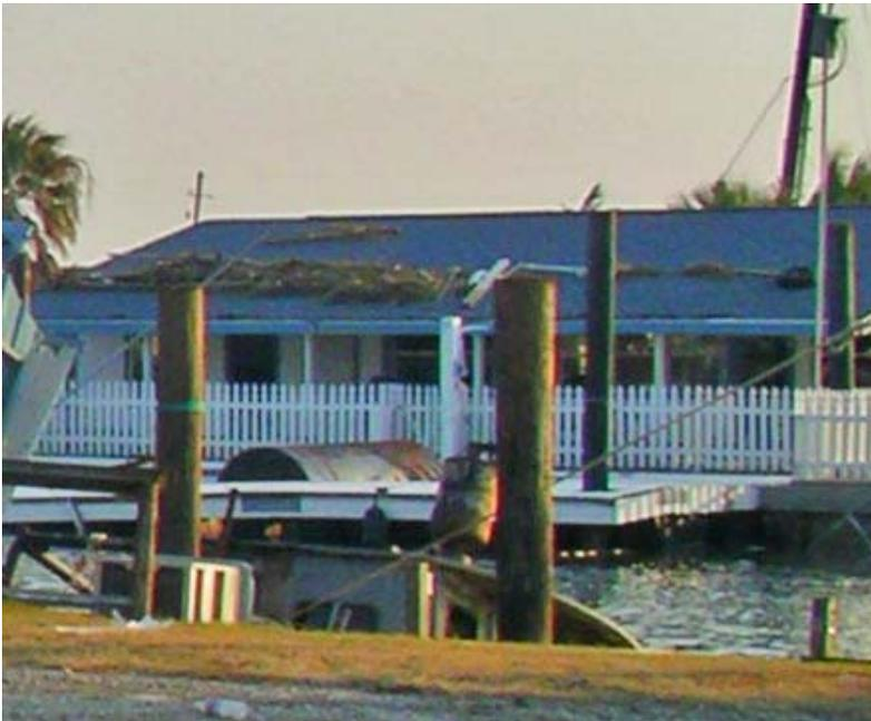
Figure 6. Surviving at-grade house less than 100m from gauge GAL-2 on the GIWW. Note debris lines on roof showing the extent of inundation, and the survival of a presumably flimsy picket fence. Maximum wave heights here were approximately 0.2-0.5m.
