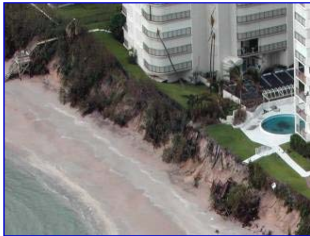
Figure 1. Beach front erosion on Hutchinson Island, FL resulting from 2004 Hurricanes Jeanne and Francis.
